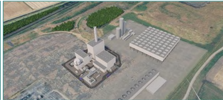
SSE Thermal, Keadby 3
